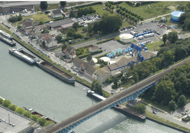
Aqualia serves more than 90,000 inhabitants in the Ile-de-France region.
