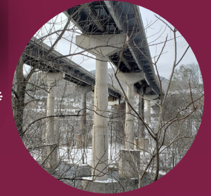
Lehigh River Bridge
