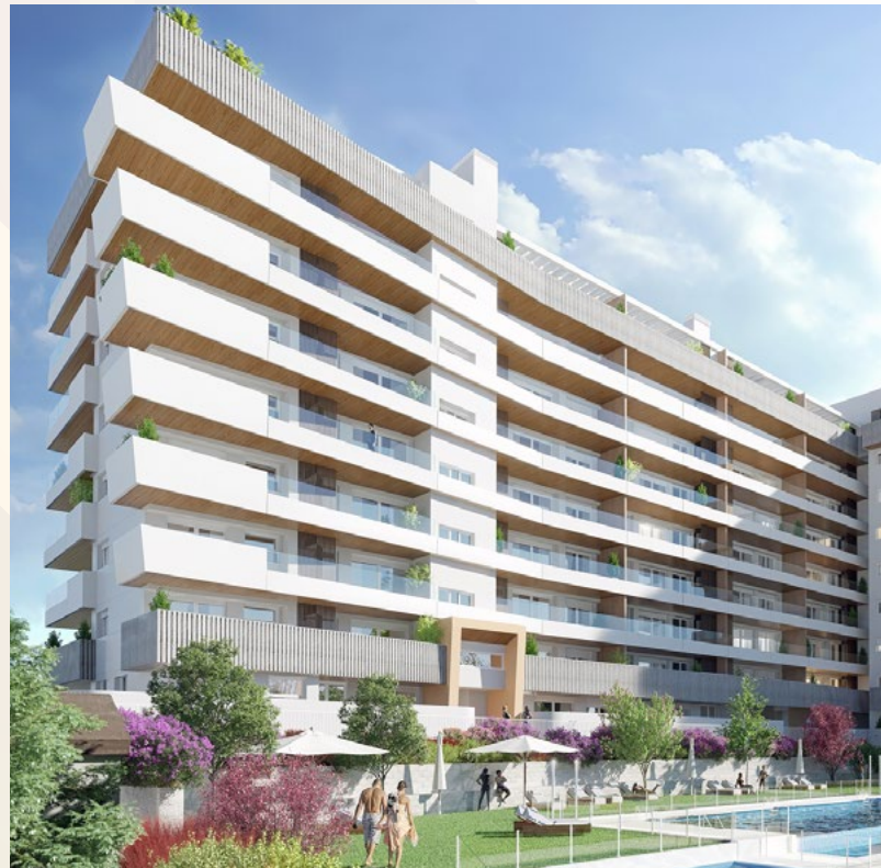
Residential building in Tres Cantos, Madrid.
